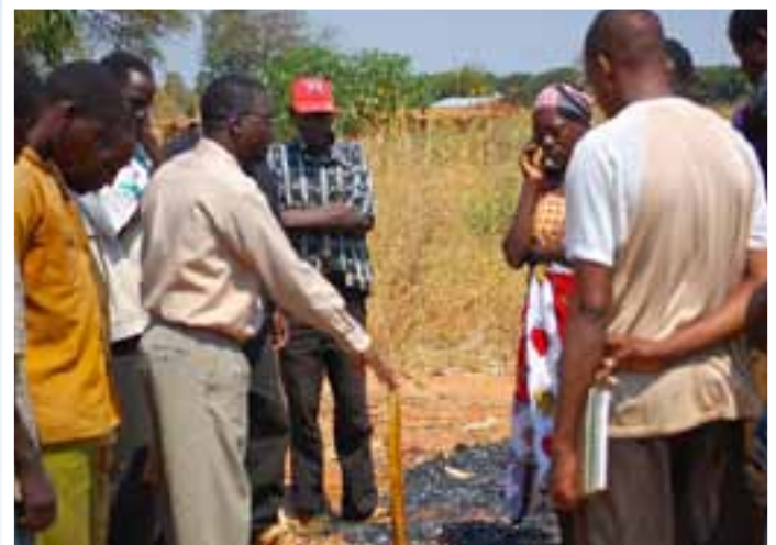
Rev. Emmanuel Petro of the Diocese of Central Tanganyika blesses the site where the Tinai water tank will be constructed.
