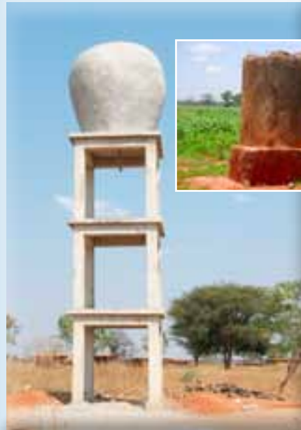
The old well tank and the newly-constructed water tank
